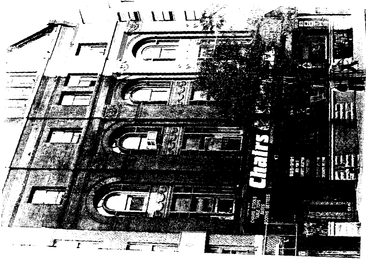
Detail of floors one through four Photo: Joseph Brooks, 1998
